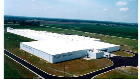
The Austin Company designed, engineered and constructed the plant and related facilities, including the freezer system; systems for unloading, storage and distribution of raw materials; and the wastewater treatment system.
